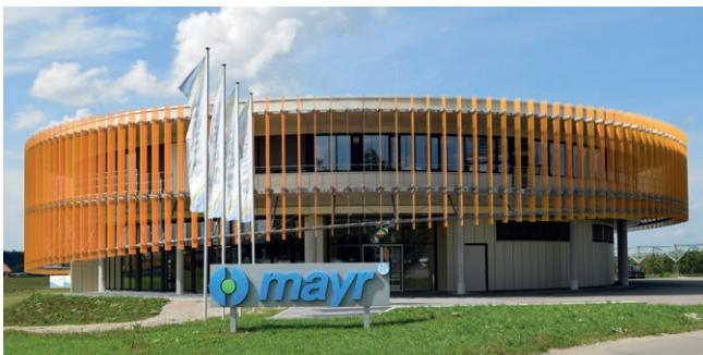
Communications Centre mayr.com – opened in 2018.
